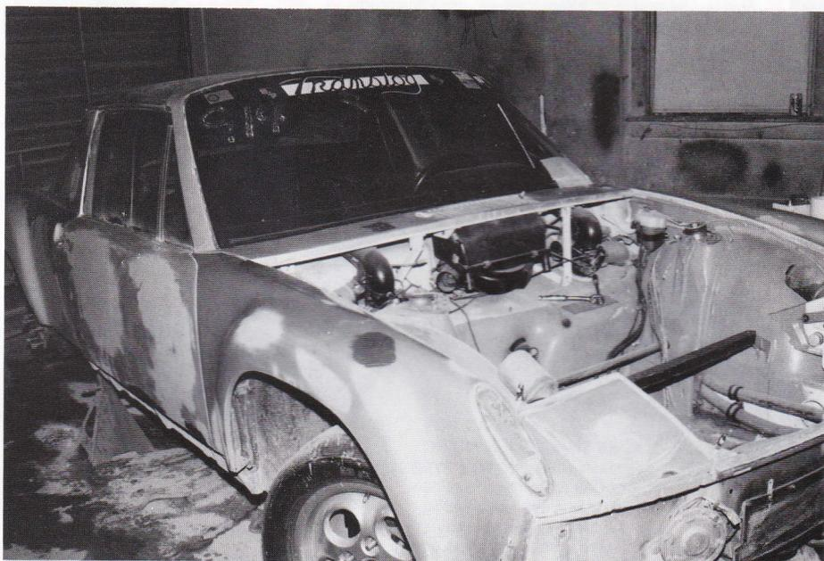
*The speedy restoration: Sunoco orange paint chips were plentiful for matching, but only one original yellow chip was found beneath the windshield wiper mechanism.*
