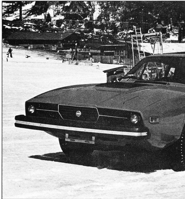
Low-speed winter capability of the various drivetrain configurations was tested at the Goldmine ski area, Big Bear, Calif. Each car was accelerated from rest on a flat section up a slope with an incline of 7-10%; the fwd Sonnet performed best.
